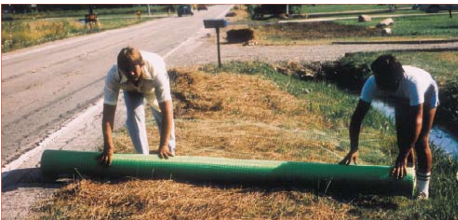
Tenax Radix being used to control straw from blowing
